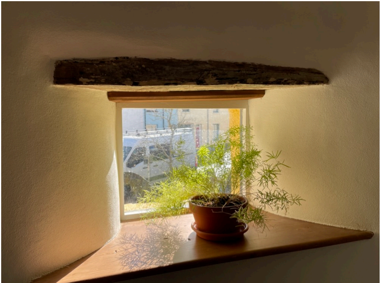
The Small window at the top of the stairs with exposed original lintel.
