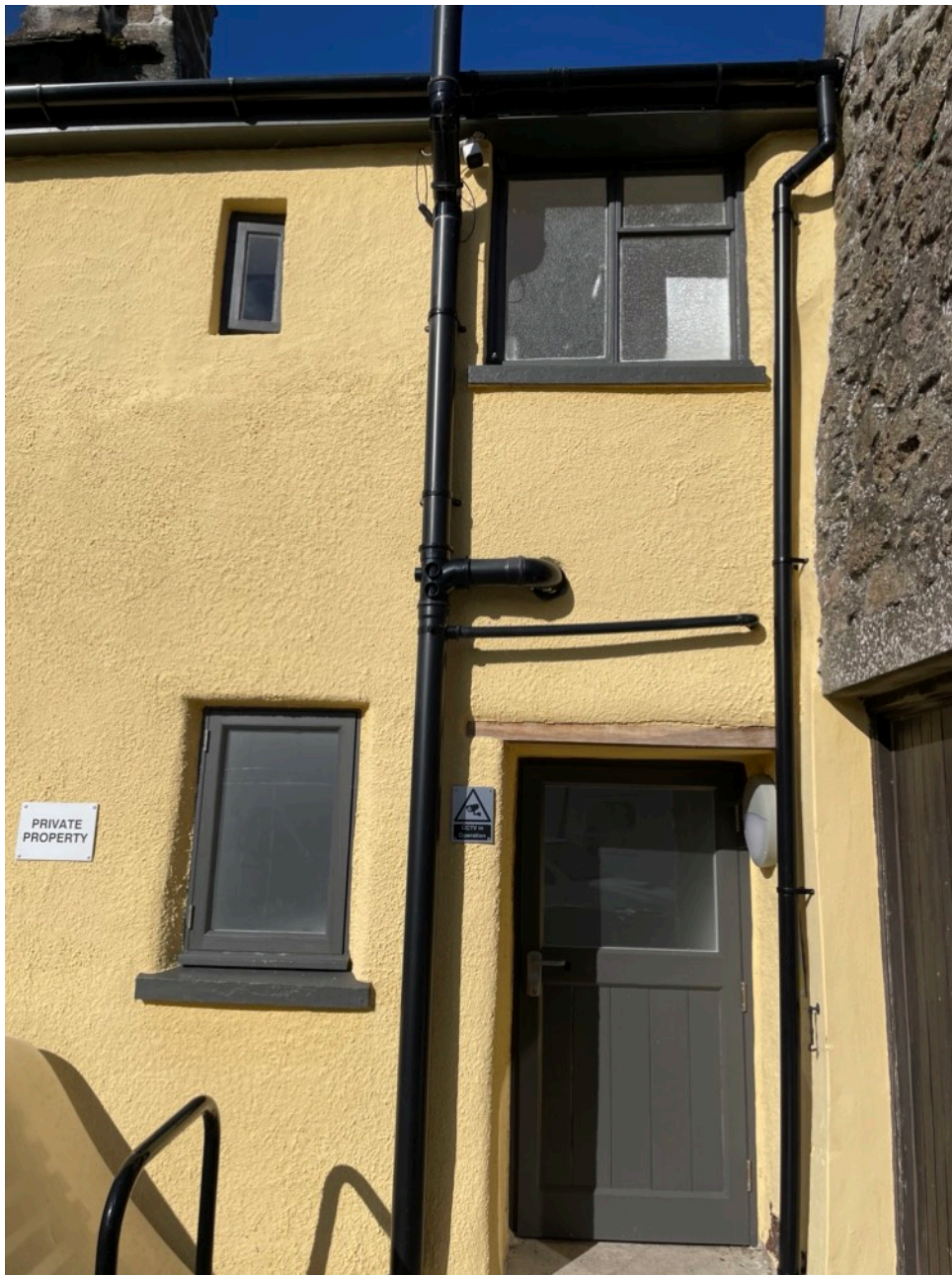
Rear of 3 Court Street, the lintel over door replaced with oak beam, guttering replaced.
