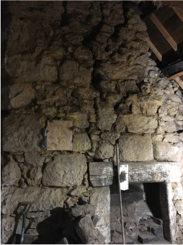
The chimney will be repaired and pointed ready for lime plastering.
