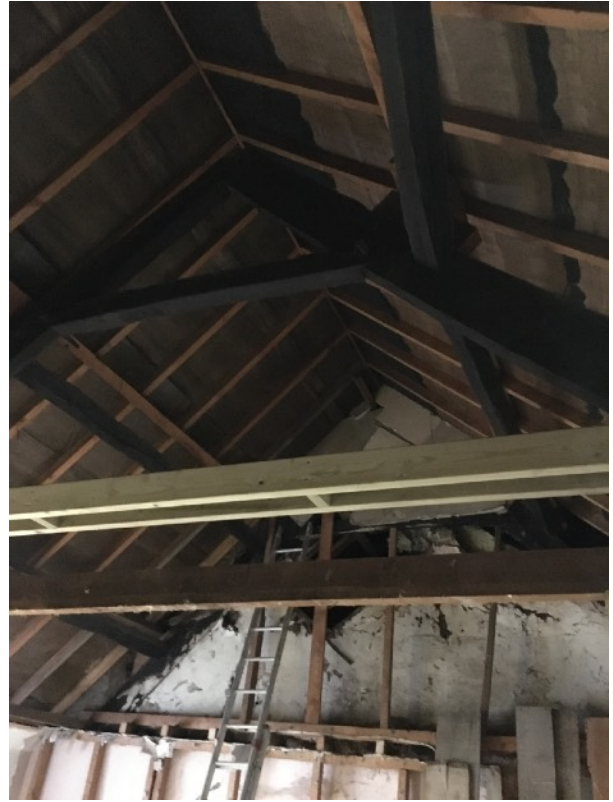
The roof needed supporting whilst repairs were done.
