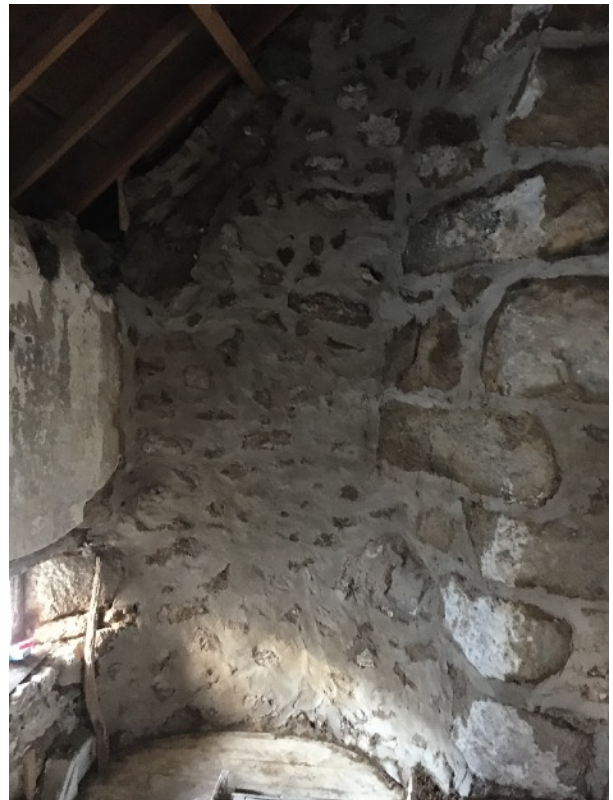
Top of stairs repointed ready for lime plastering.
